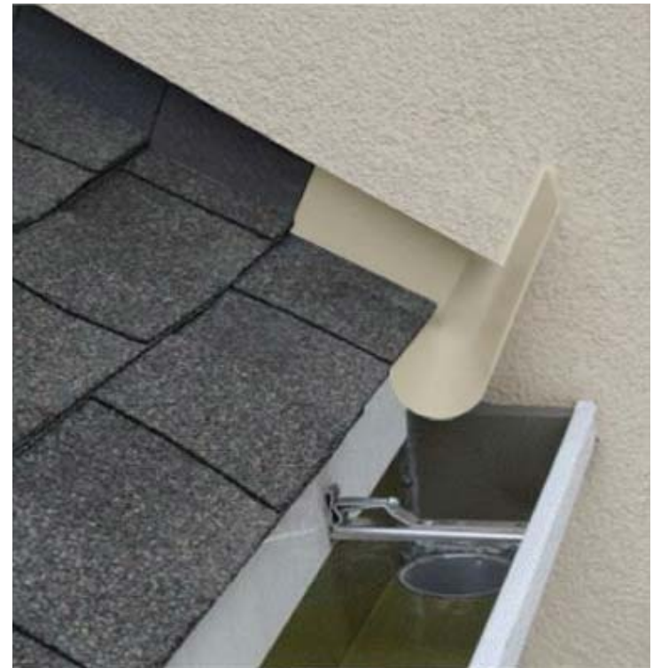
Kickout Flashing
