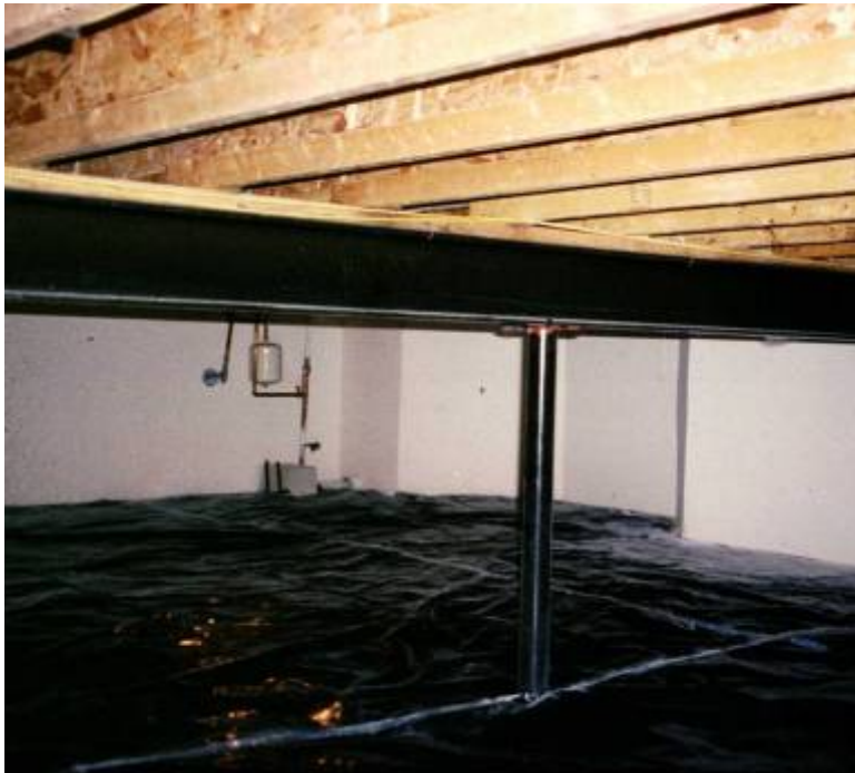
CRAWLSPACE VAPOR AND RADON BARRIER
