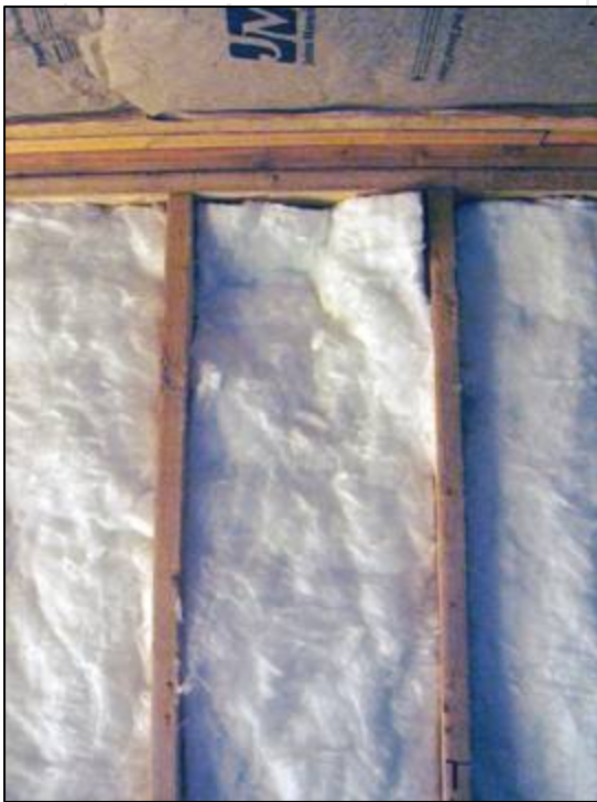
Sound insulation in place.
