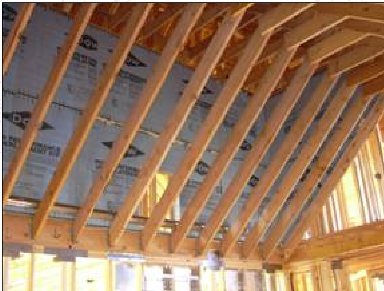
Kneewall Open to Attic Rafters
