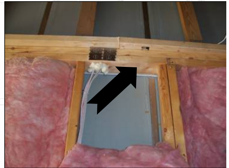
The wire hole is sealed, but the party wall isn't.
