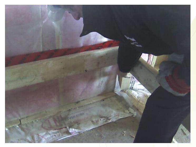
Air barrier is mechanically fastened behind the tub although the side were missed.
