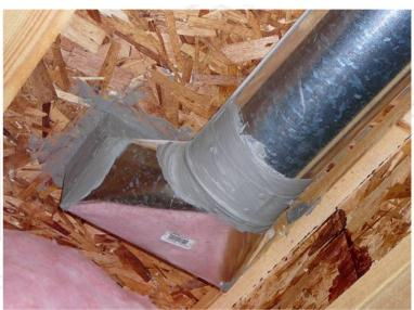
DUCT BOOTS & SEAMS SEALED WITH MASTIC
