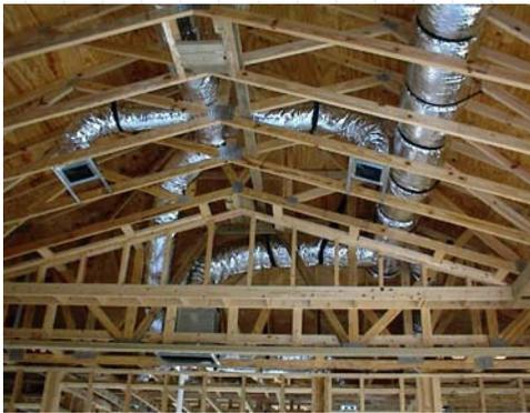
Ducts located in the unconditioned space also have a heat gain that adds to the cooling load of the building.
