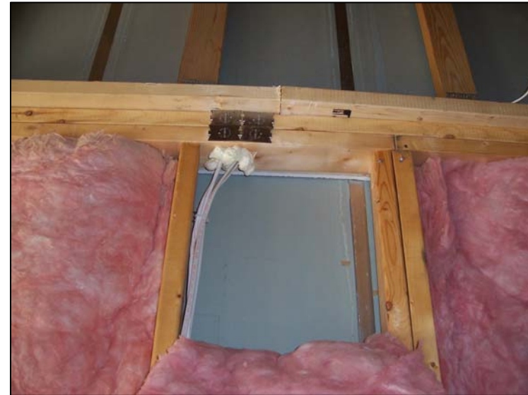
Wire hole sealed, but party wall is not
