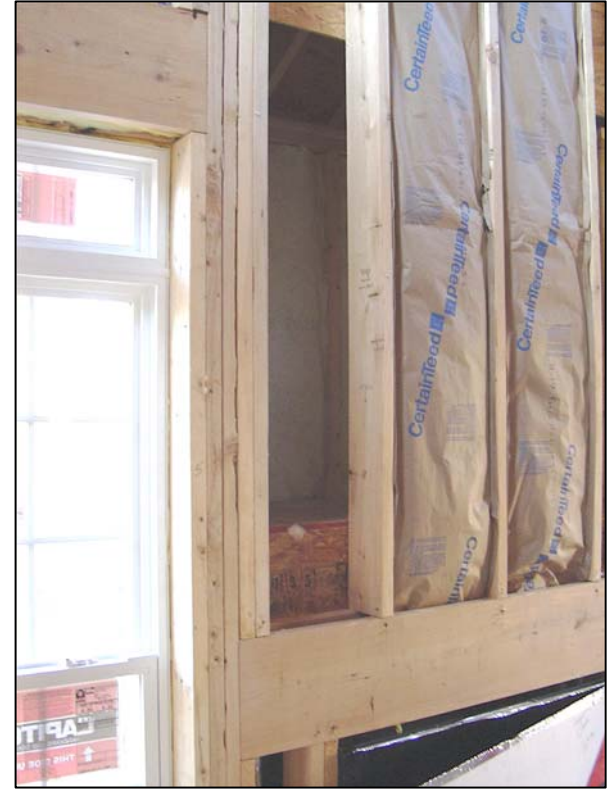
Insulation in wrong place, area not sealed
