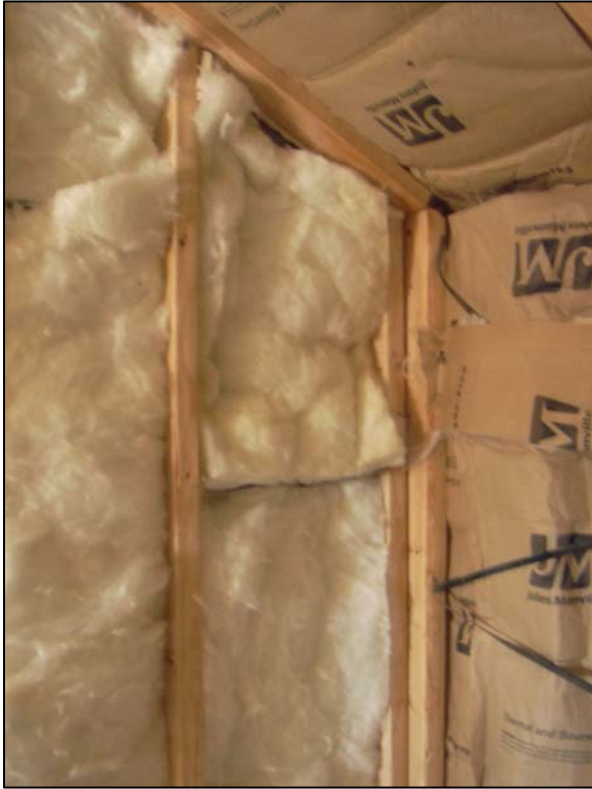
Insulation in place
