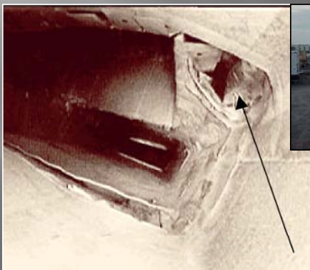
View at plenum – note large hole
