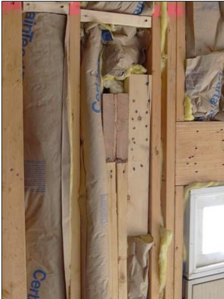
Insulation in place.
