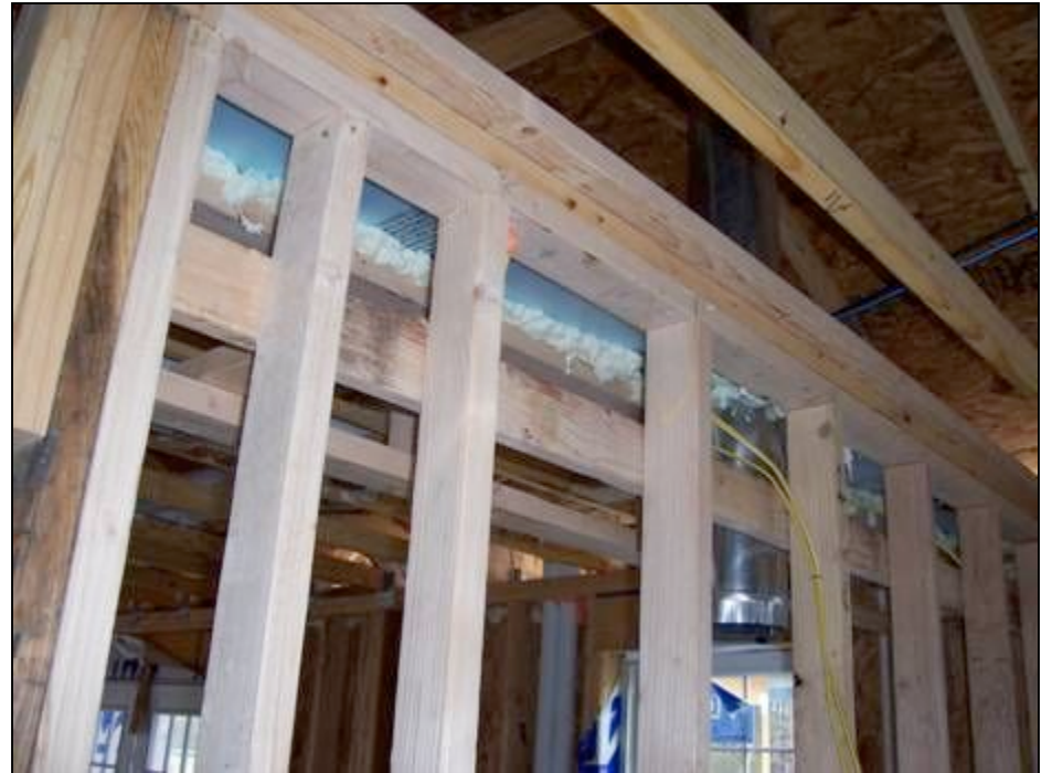
Kitchen soffit sealed with styrofoam and foam.
