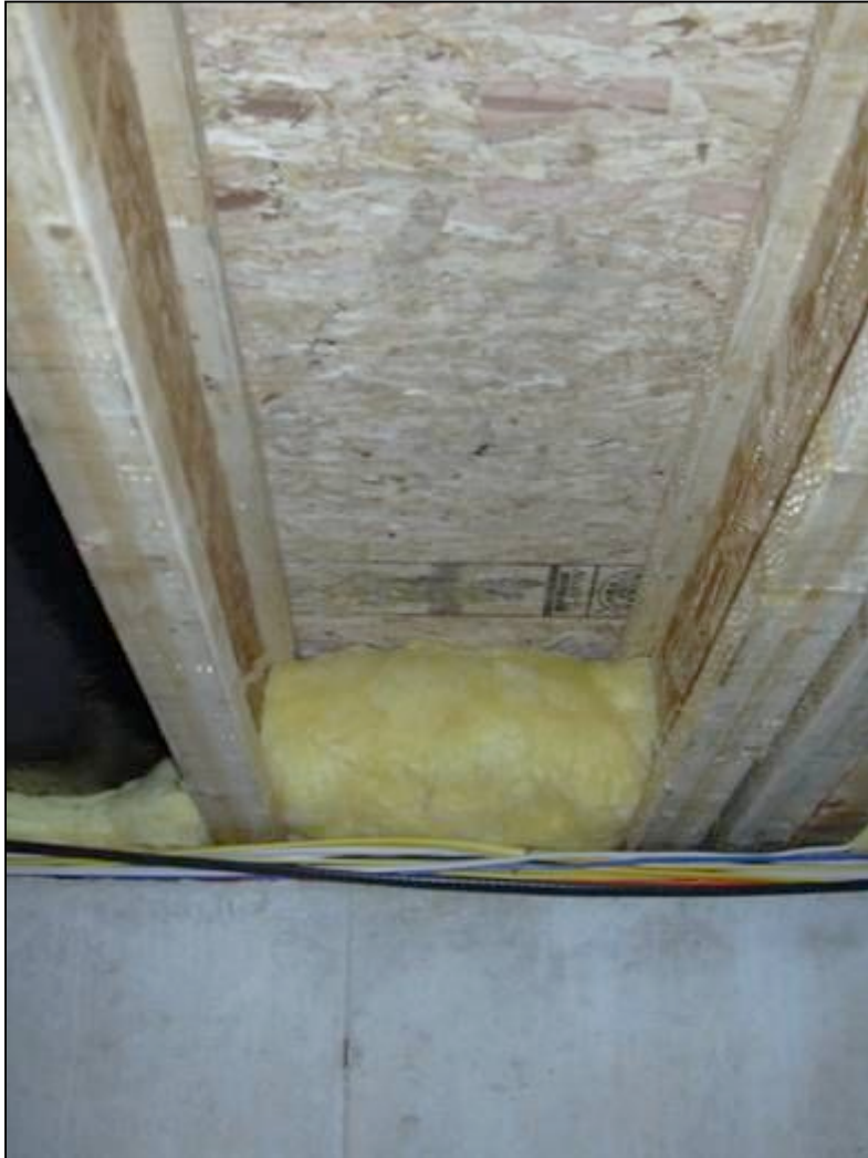
Insulation - full depth of floor joist.
