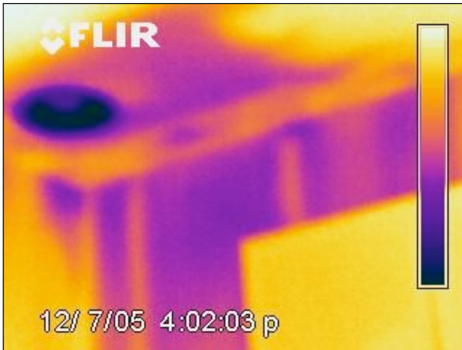
Chase open from attic into interior wall.
