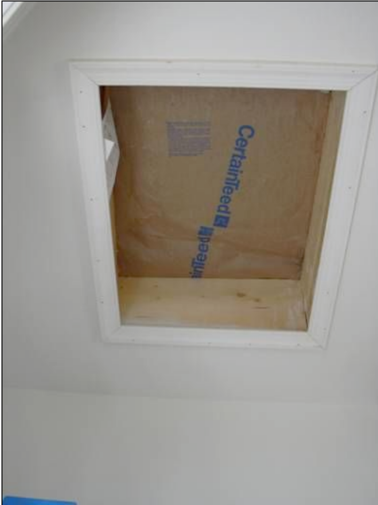
Wrong way to insulate - air barrier and insulation not aligned.
