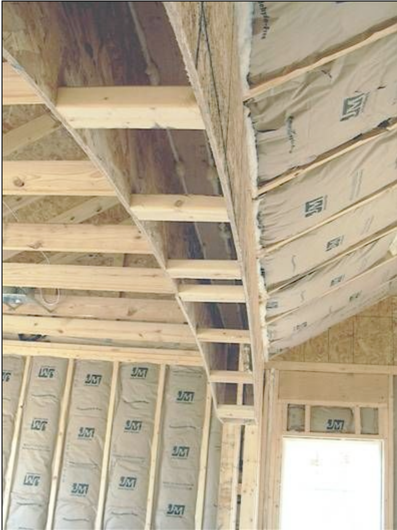
Archway between 2 rooms forming 'soffit' - sealed inside with foam.
