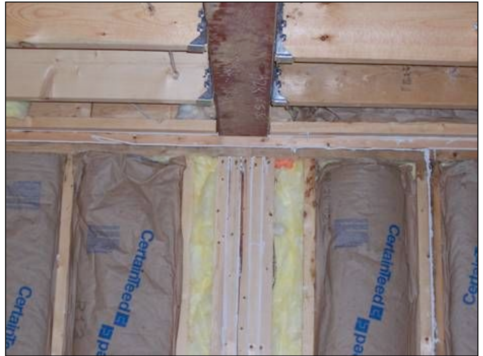
Caulk where not necessary. Wasted time and money.
