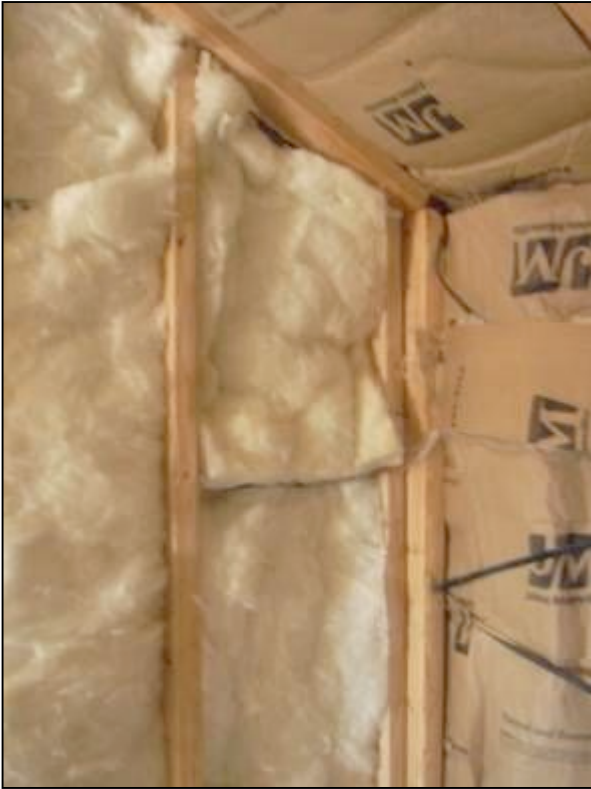
Insulation in place.
