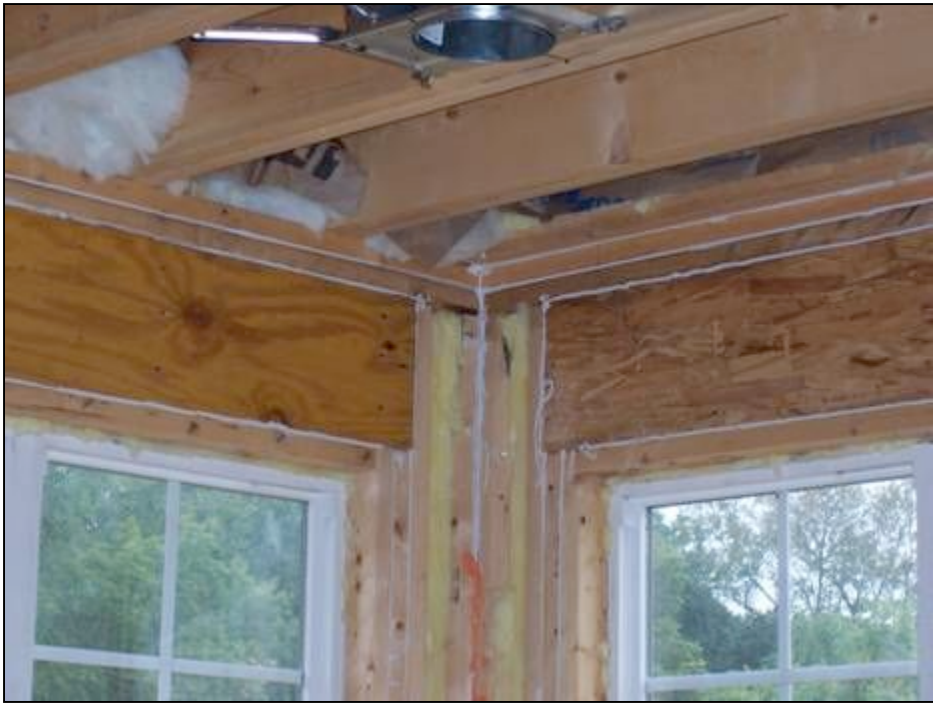
Caulk where not necessary.
