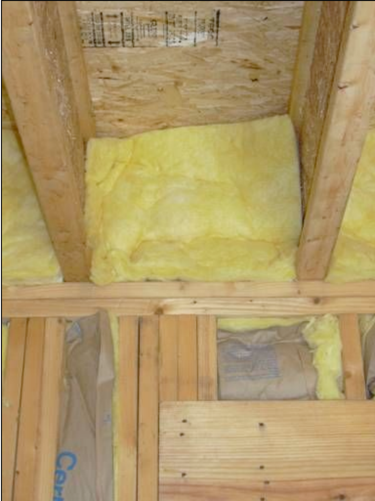
Insulation in place.
