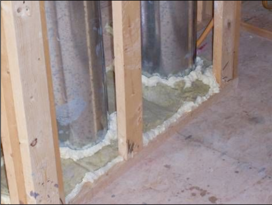
Airtight foam on pervious rock wool.
