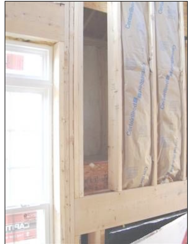
Fireplace not sealed, insulation in the wrong place.
