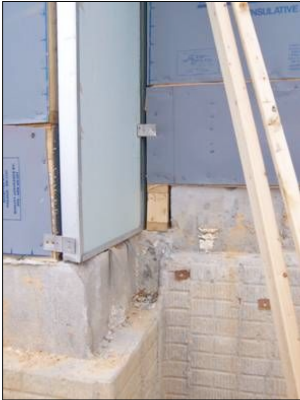
From the outside, corner between 2 units will get covered by 'J' channel siding, but will still leak air.
