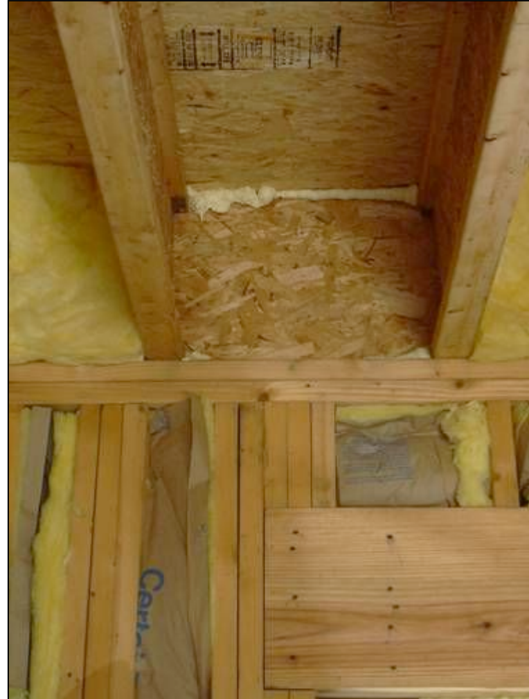
Band joist between floors sealed.
