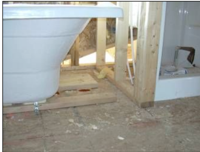
Tub and shower open to attic behind.
