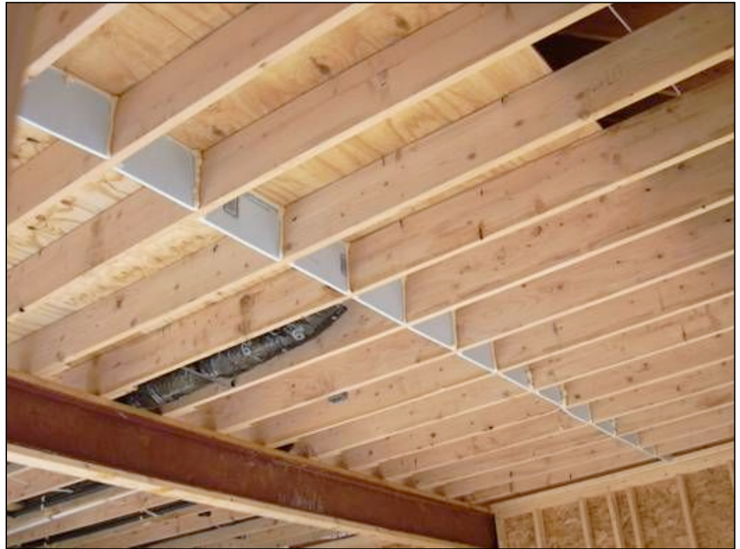
Air dams under exterior wall of room above garage
