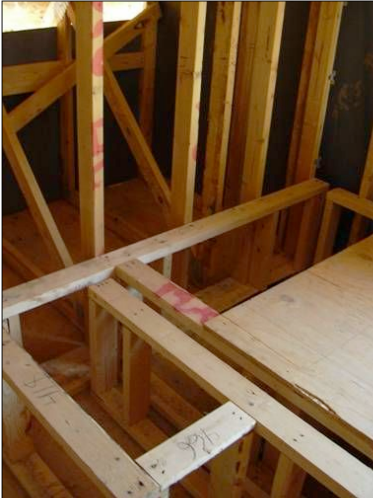
Soaking tub base open to knee wall attic
