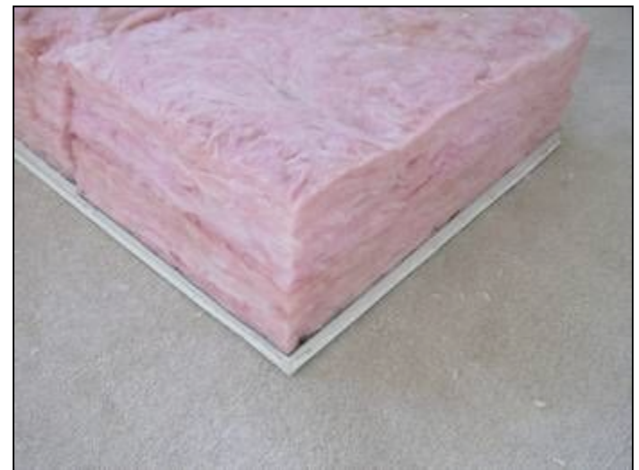
Insulation installed to edge of hatch cover.
