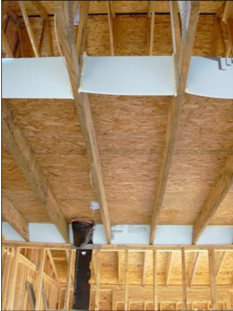
Air dams at both ends of open joists under room over garage
