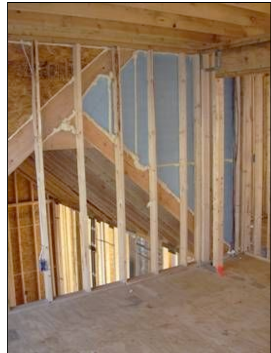
Kneewall Covered at Attic, Not Heated Space
