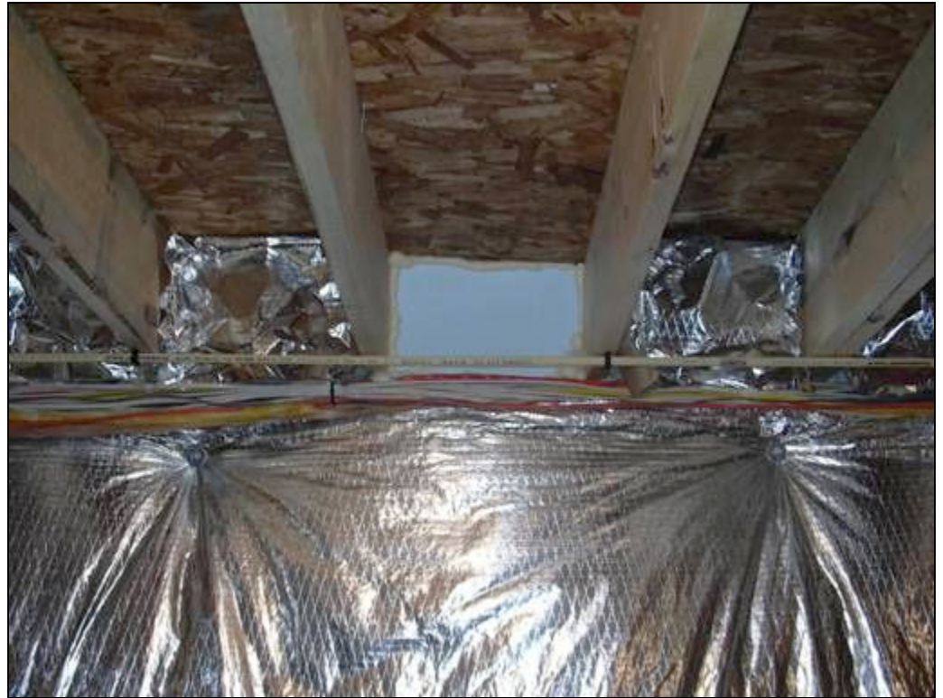
Alternative - overhang sealed and insulated first, then air dam sealed tight. In small overhangs, this tends to make floor colder.
