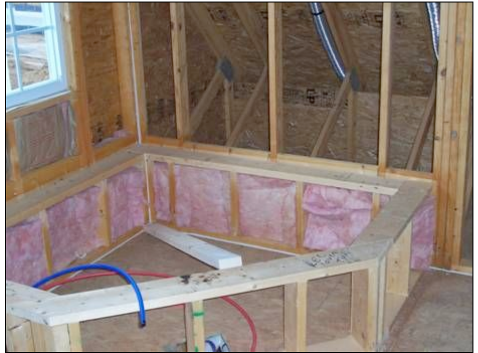
Plenty of caulk, but no airtight back on insulation in attic.
