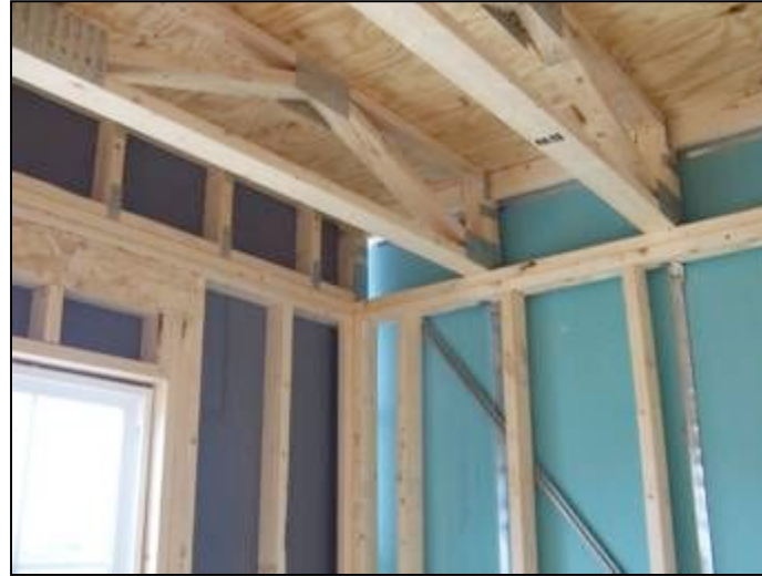
Area at band is just as important as the wall itself
