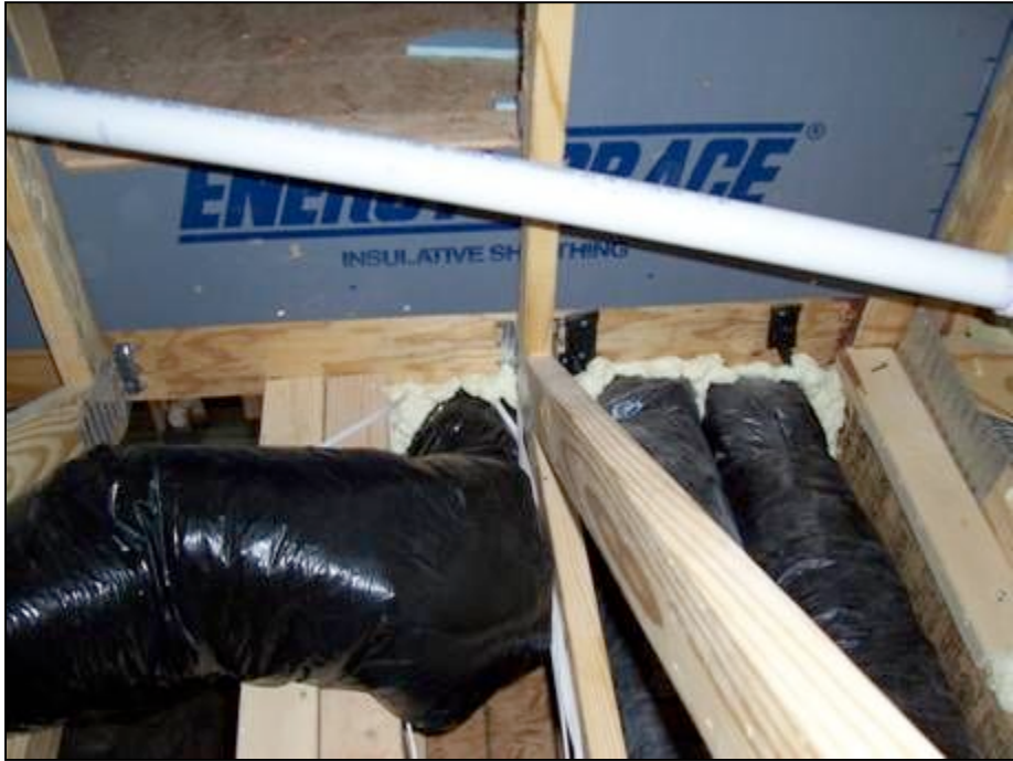
Tightly sealed ductwork.
