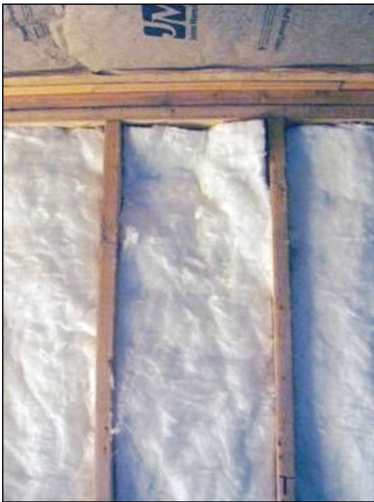
Sound insulation in place.
