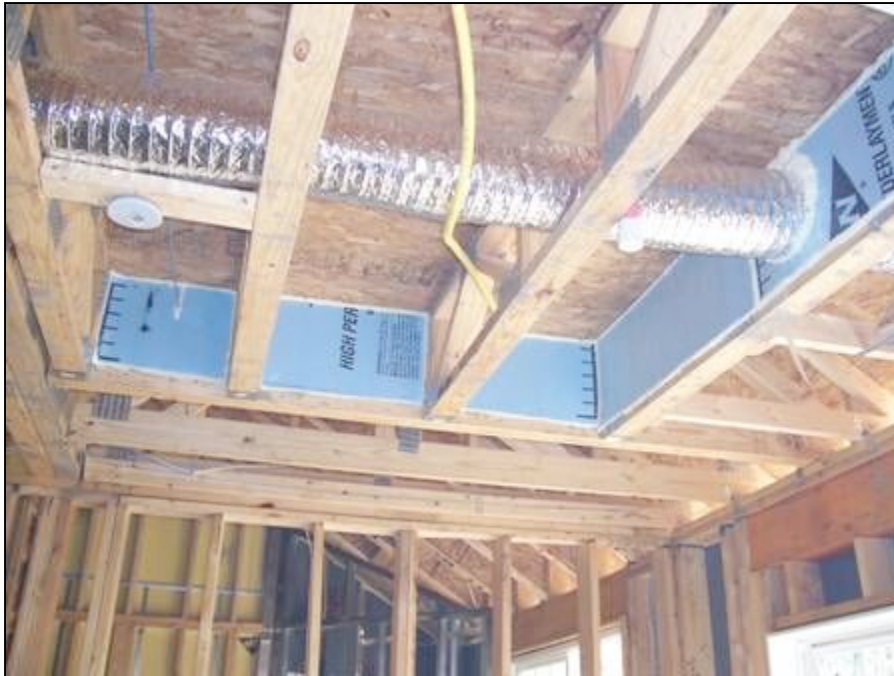
Joist cavity open to attic on 2 sides - sealed tight.
