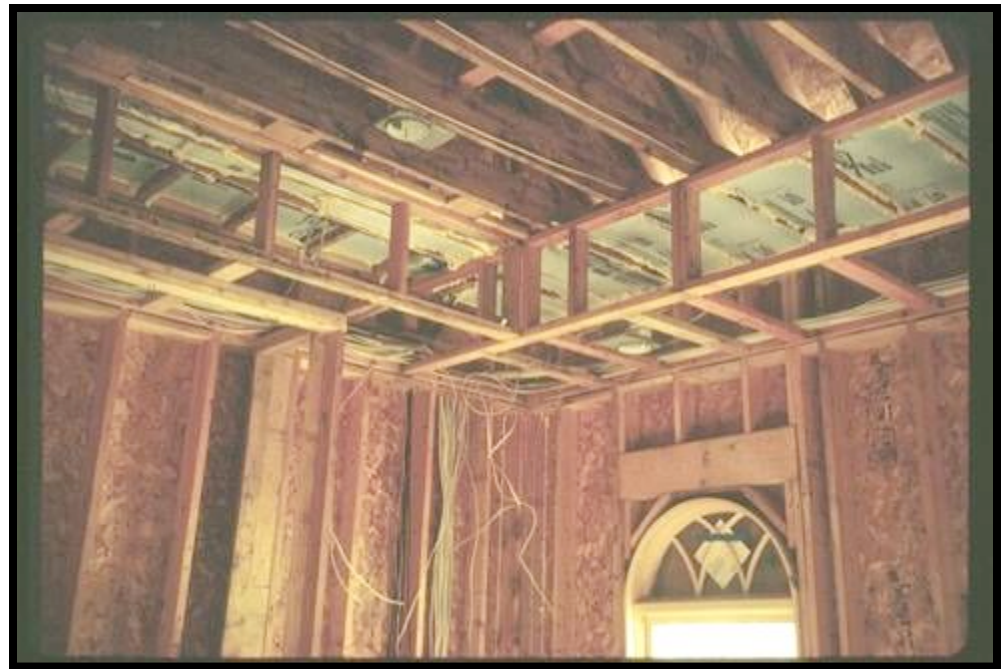
Kitchen soffit sealed at joist level with styrofoam & foam.
