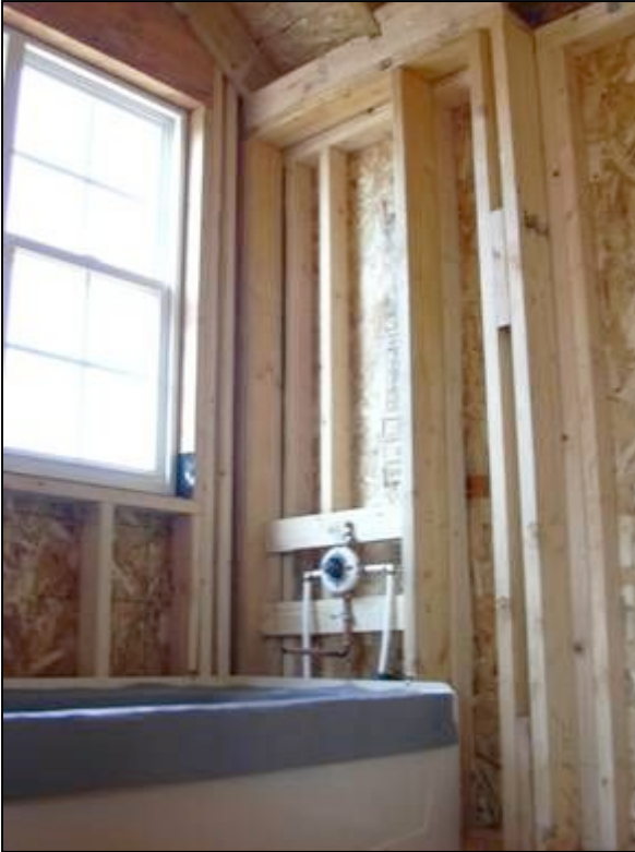
Packed out wall at head of tub open to attic.
