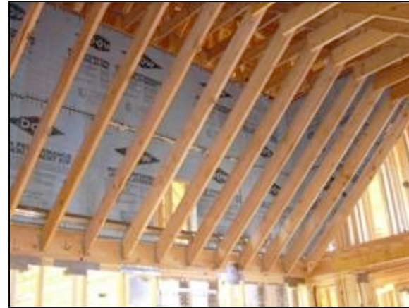
Kneewall Open to Attic Rafters
