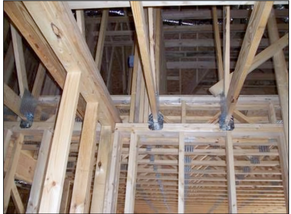
Looking from an attic kneewall into joist cavity.
