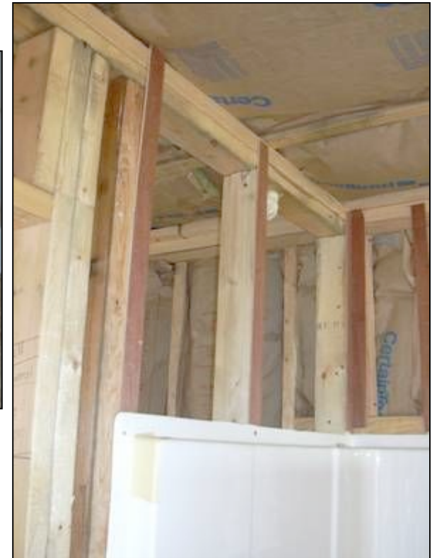
1/4" strips added to make sheetrock line up with tub flange – 1/4" slot at top of wall.
