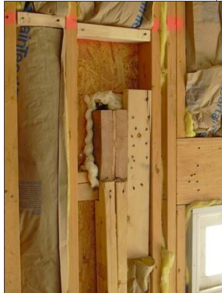
End of front porch beam sealed.
