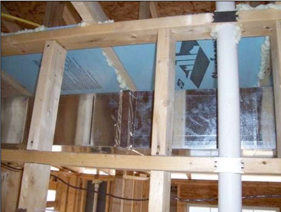
Duct soffit sealed with styrofoam and foam.
