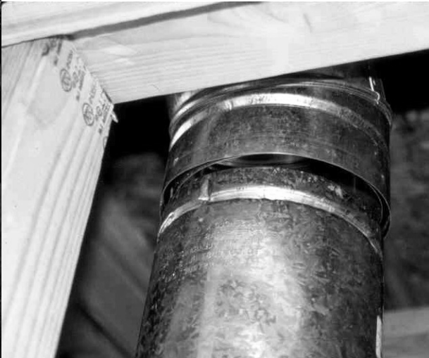
This is from a new home!
