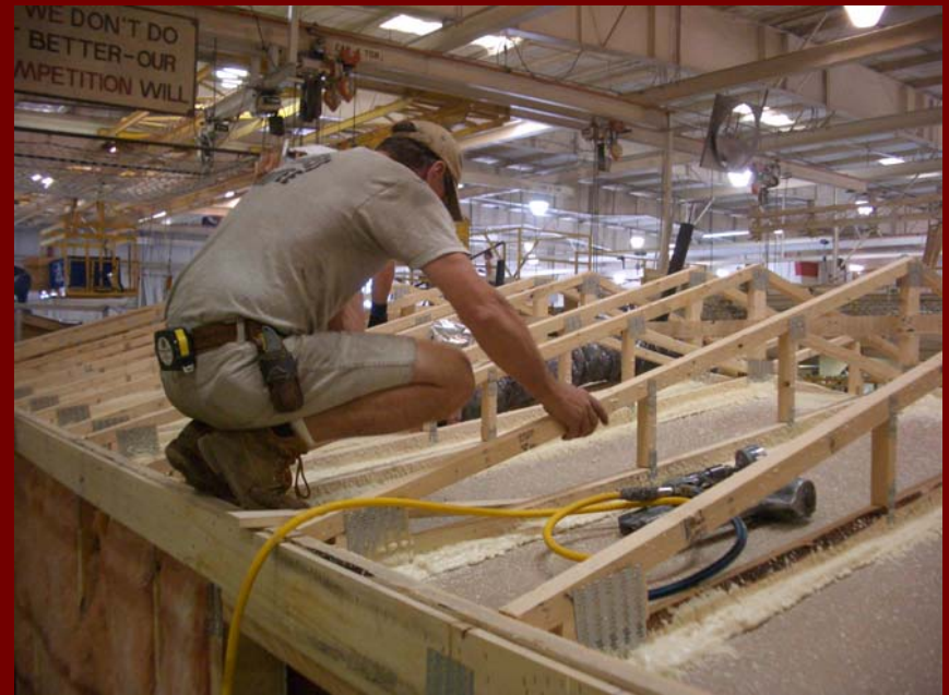
Ceiling drywall is foamed to roof trusses
