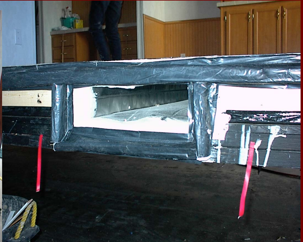
Factory-installed marriage line gasket for through-the-rim crossover
