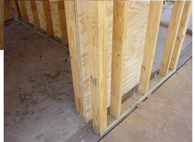
**Low cost wood frame Safe Room (not FEMA standard) with separate framing and ceiling, pocket for sliding impact door – for hurricane and mild tornado resistance**
