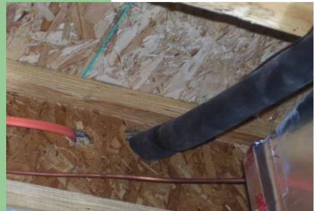
Rim Joist / Return
