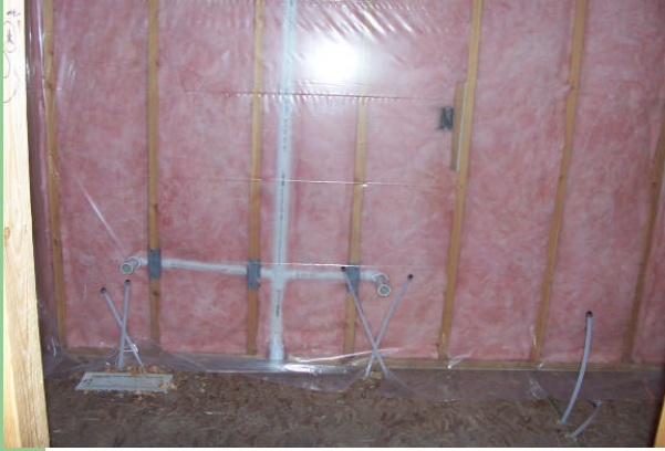
Splitting of Batts
