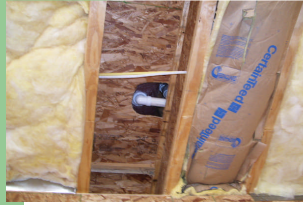
Framed Floor Above Garage
