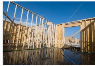
Traditional Site Built
