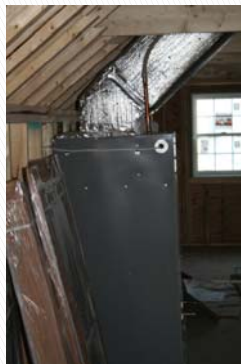
Air handler located in unconditioned attic...disconnected ductwork
