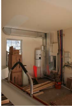
Connection between basement, apartment, bonus room, and attic...
