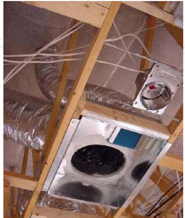
DUCTED FRESH AIR SUPPLY
