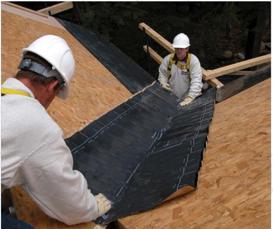
BITUMINOUS MEMBRANE AT VALLEYS
