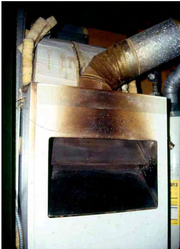
Combustion spillage
