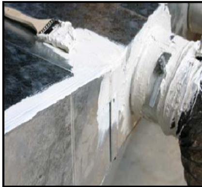
Recommended: Seal all duct connections with mastic
