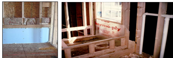
Two installations of air barriers at tubs adjoining exterior walls
